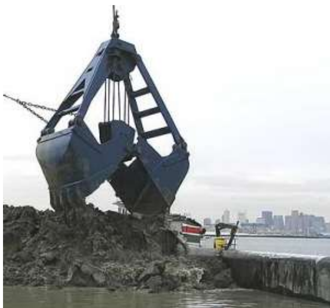
Figure 7 – On the left, a mechanical bucket dredging showing consolidated material, and on the right, the hopper of a dredge showing a slurry of dredged material Sources: Norfolk Dredging Inc. and Seaturtle.org.
